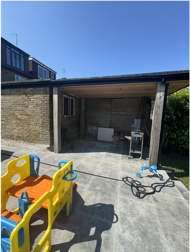
B - Existing Garage Extension
